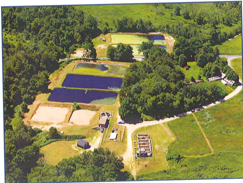
Existing WWTP Site
